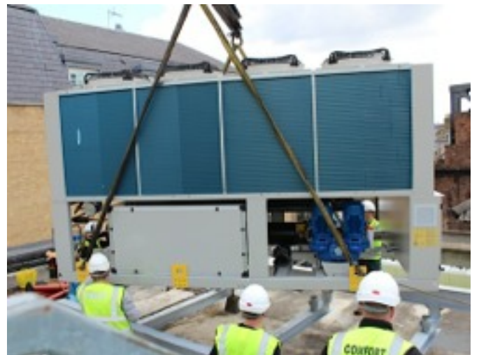
New Daikin chiller lifted in to position
